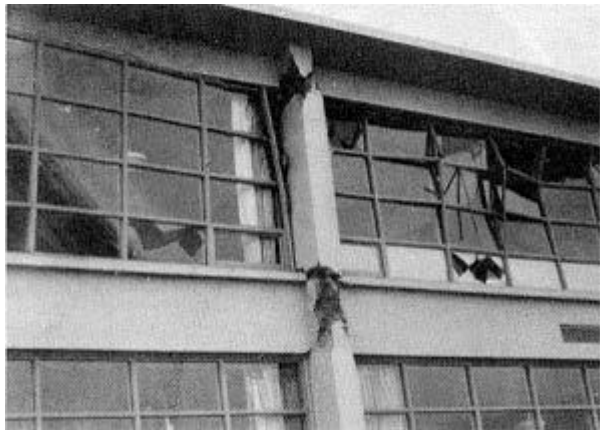
Obvious damage to primary structural elements, severe cracking of walls, or other signs of severe distress Condition: UNSAFE
